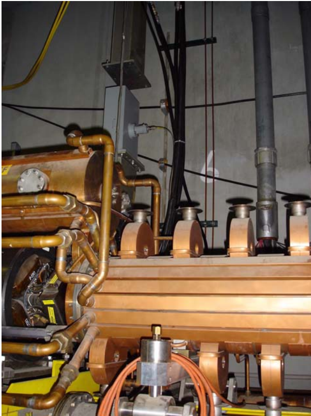
Drive through type N transition on waveguide
