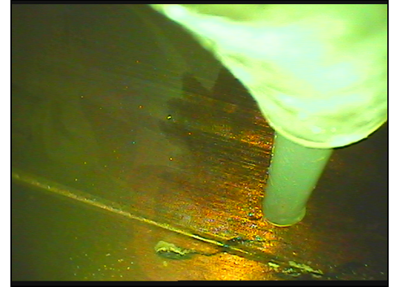
Tygon tubing with poly-flow working tool working at the bottom of cell #8
