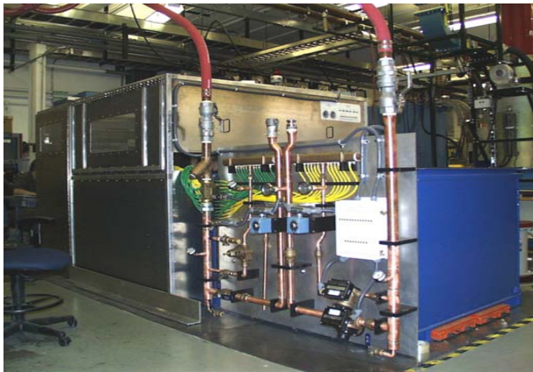
HIGH VOLTAGE CONVERTER MODULATOR
