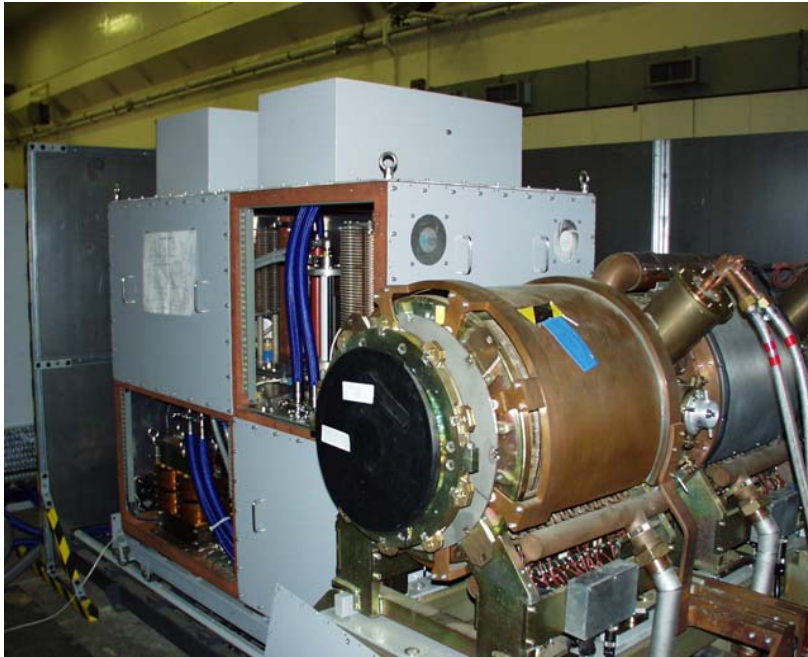
RF amplifier connected to cavity
