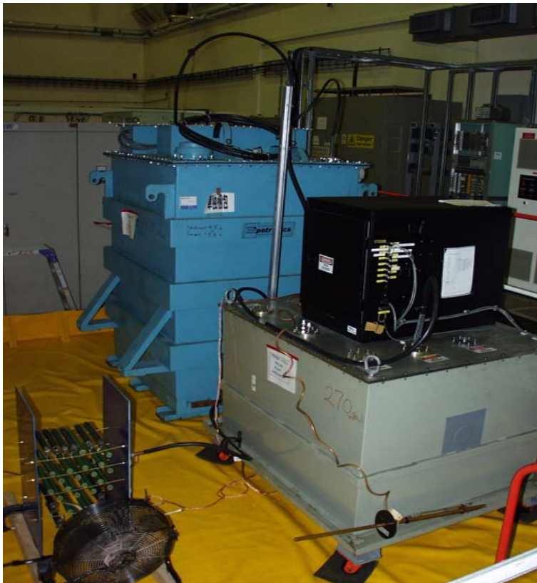
T-R set (blue) and Buck Regulator/Fast Switch tank
