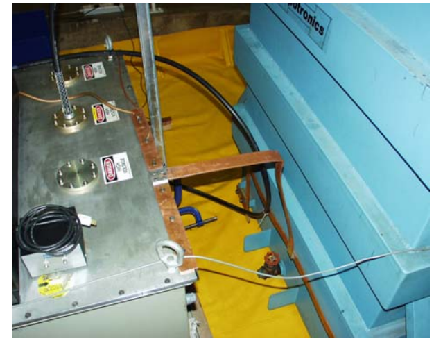
Installation of adequate bonding conductors between sub-systems
