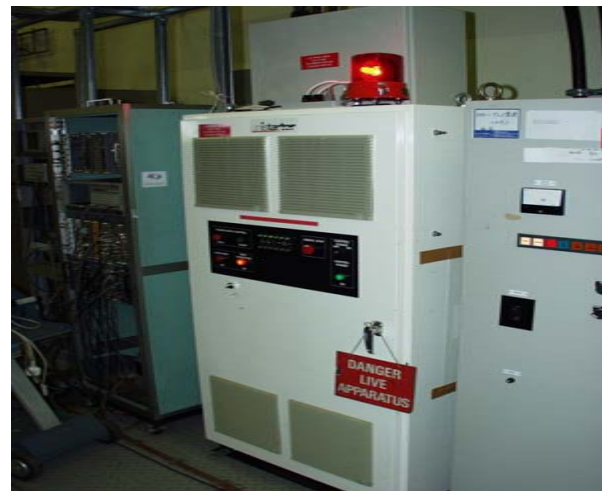
Installation of step-start in T-R set primary power feed
