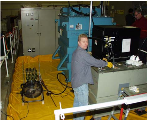
Filling Buck Regulator/Fast Switch tank with Midel oil
