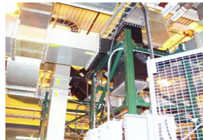
Four-Port Waveguide Switch.
