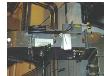
1 MW CW RF Power Test of Waveguide Shutter in Closed State.
