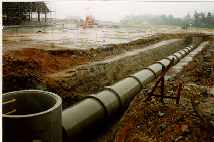
Fig. 11. Drain pipe before tunnel floor construction.
