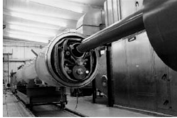
Figure 10: Cold mass connected to the vacuum vessel
