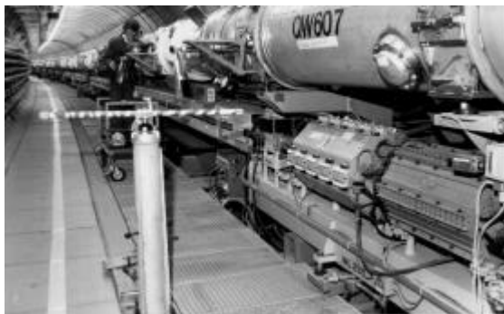
Figure 27: Prealignment with respect to the tunnel traverse
